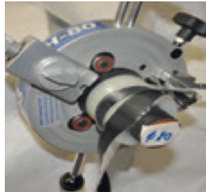
peeling the semicon layer
